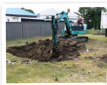
Excavation of the site
