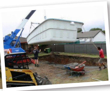
Crane used to place pool
