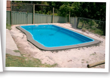
Concrete Bond Beam
